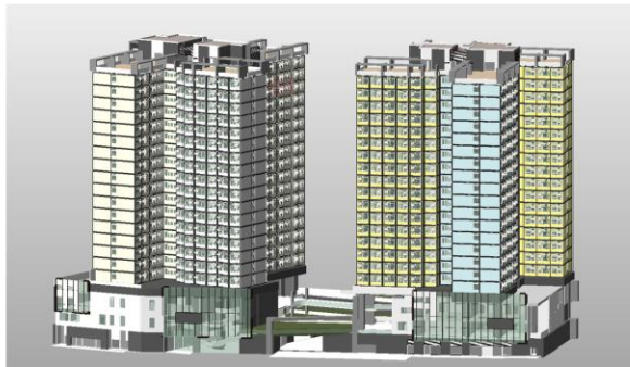
(b) Overall view of HKU's WCH Student Residence project
