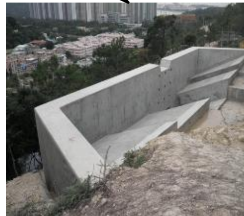
Rigid debris-resisting barrier
