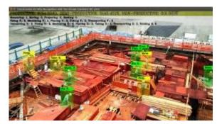
Pi is non-intrusive and requires little additional cost in its implementation since surveillance cameras are commonly used in construction sites. Thus, it can be easily extended to improve construction safety management. It can conduct site inspections and make records so as to lessen the workload of human inspectors.
